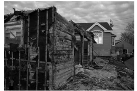
| Route Kennedy Carrier-Station
